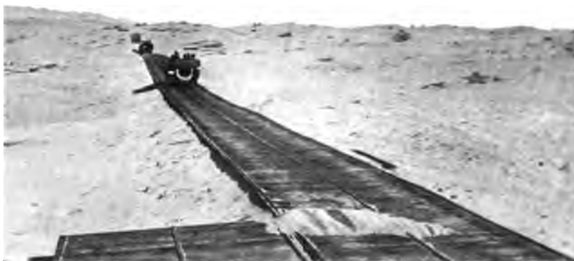
Plank road completed. Turn-out in left foreground
